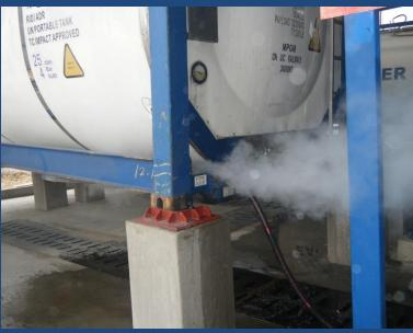
This station is where the ISO tanks interior are clean, discharging the cargo remnants, wash and dry. This station also is where the waste disposals from the tank remnants are kept and discharge in the accordance to the local health and safety requirement. Basically, the cleaning stations facilities consist and require the following:
